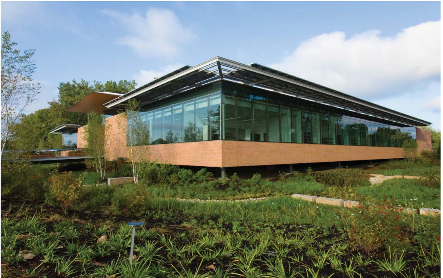
Southwest corner of building indicating building "floating" above floodplain
