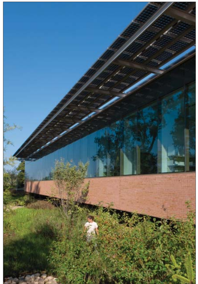
Cantilevered "brise-soleil" solar panels shade the principal investigators' offices
