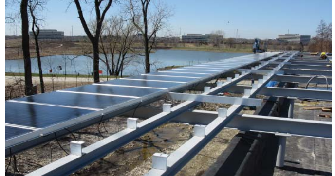
Photovoltaic cells under construction
