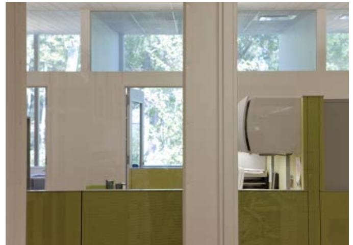
Interior clerestories allow for natural ventilation and natural light
