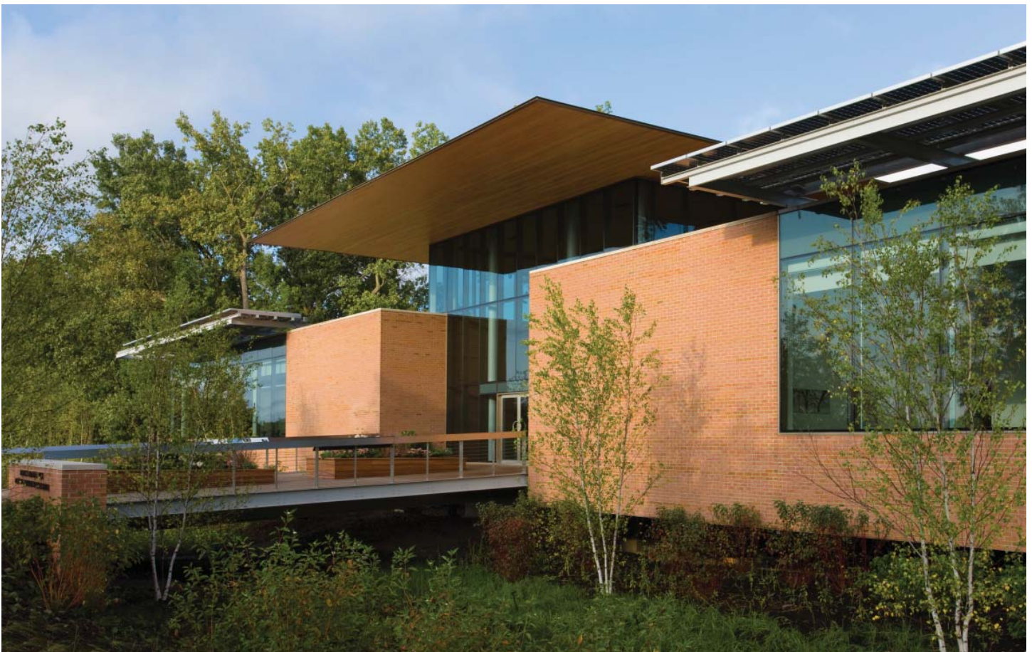
Main entrance accessed by a bridge over a rain garden
